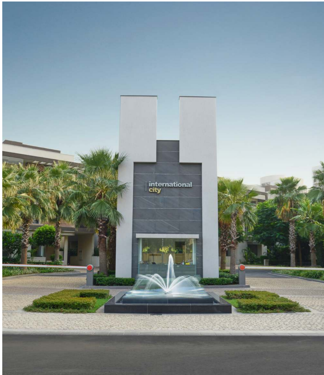
ACTUAL IMAGE OF THE BLOCK B ENTRANCE
