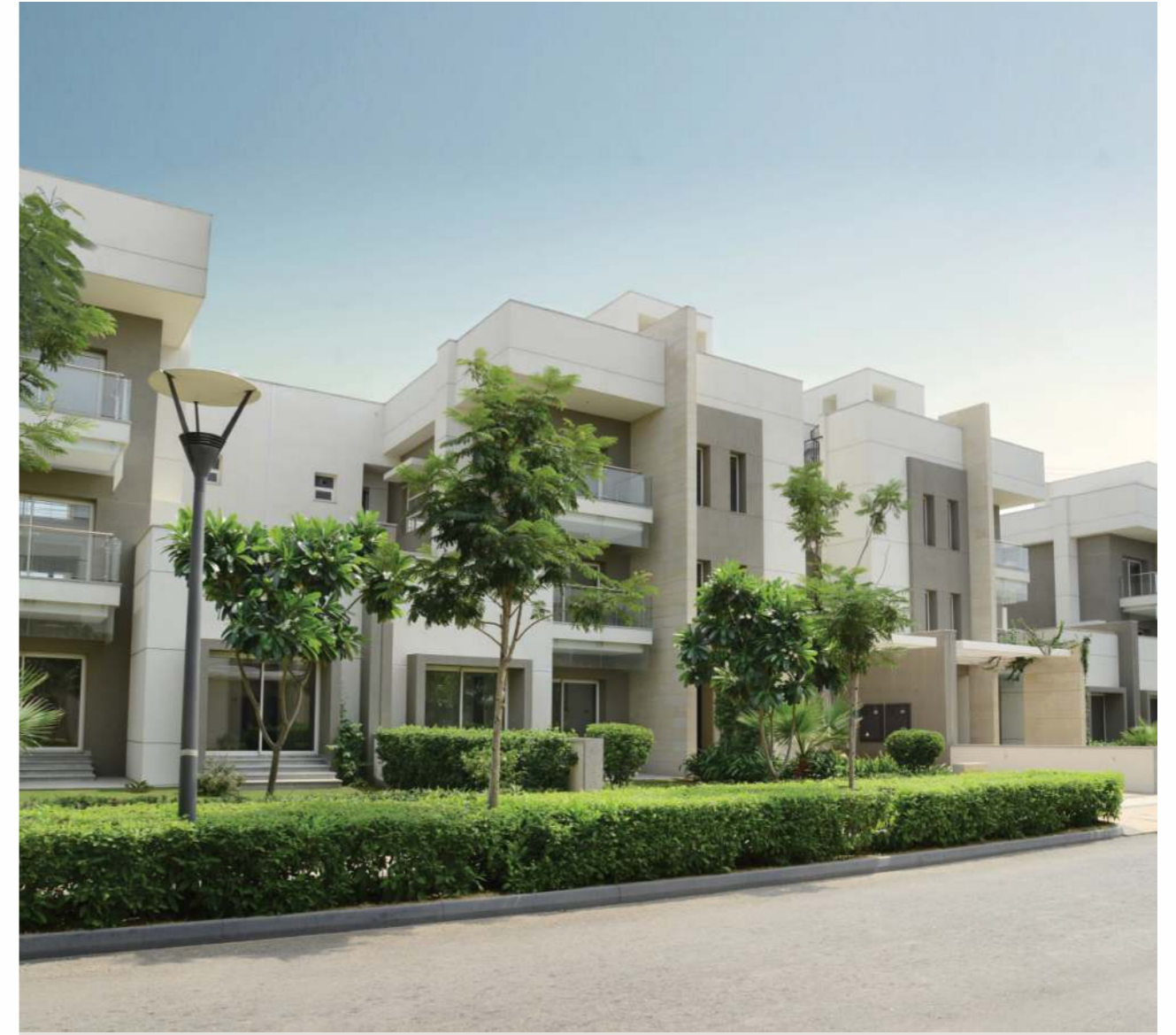
ACTUAL IMAGE OF DUPLEX VILLA, BLOCK E
