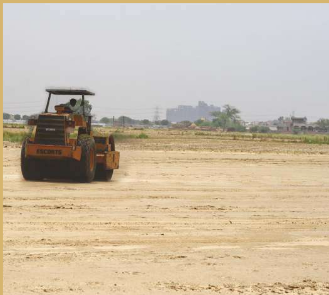
NORTHERN PERIPHERY ROAD (DWARKA EXPRESSWAY) UNDER CONSTRUCTION
